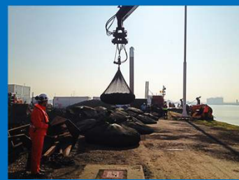
Belgium 2014 scour protection
