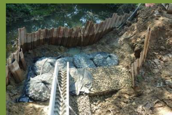
U.K. 2014 foot protection with gabion
