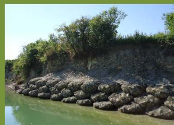
Czech Republic 2013 bank protection
