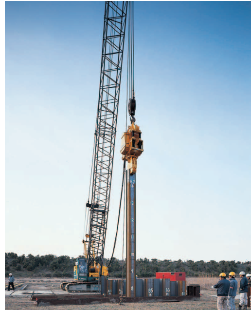
Driving of U-type sheet pile
