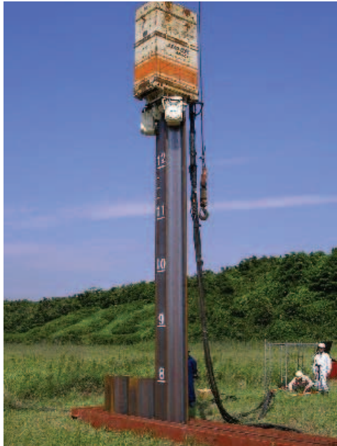
Driving of hat-type sheet pile 900
