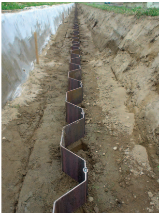
Subsurface water flow stoppage wall
