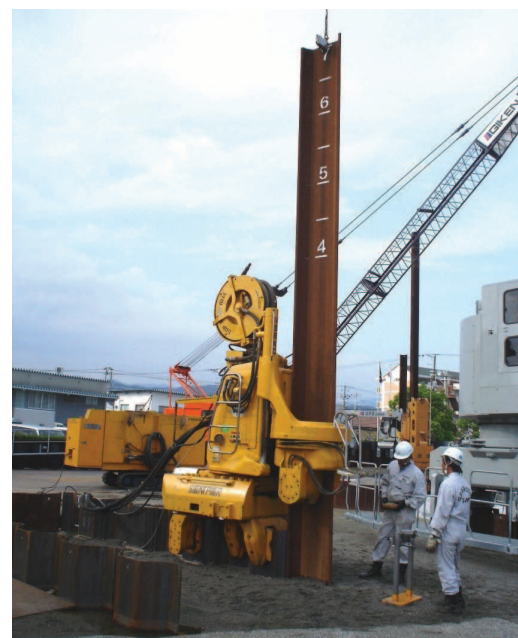
Pressing-in of U-type sheet pile
