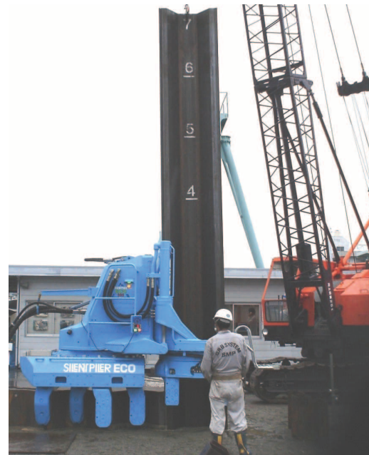
Pressing-in of hat-type sheet pile 900
