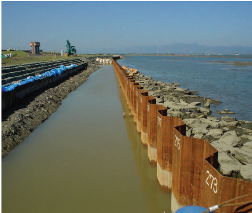
Permanent use as well as temporary cofferdam use
